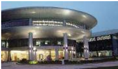
China Technology Center Shanghai, China
